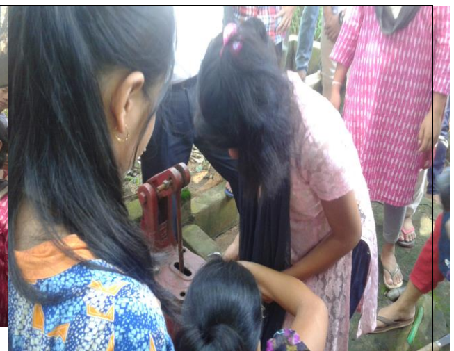
Practical exercise how to fix a tube well
